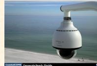
The CoastalCOMS camera installed at a Penscola Beach Florida
